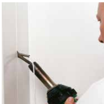
Altro Whiterock Welded joint
